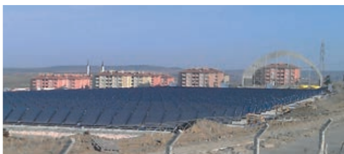
Solar district heating
