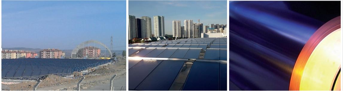
Solar thermal collectors use energy from the sun to generate heat for heating, hot water and solar cooling. This energy is free, environmentally friendly and reliable. The heart of flat-plate, air and evacuated-tube collectors is the absorber. It collects the energy in sunlight and converts it into heat.
